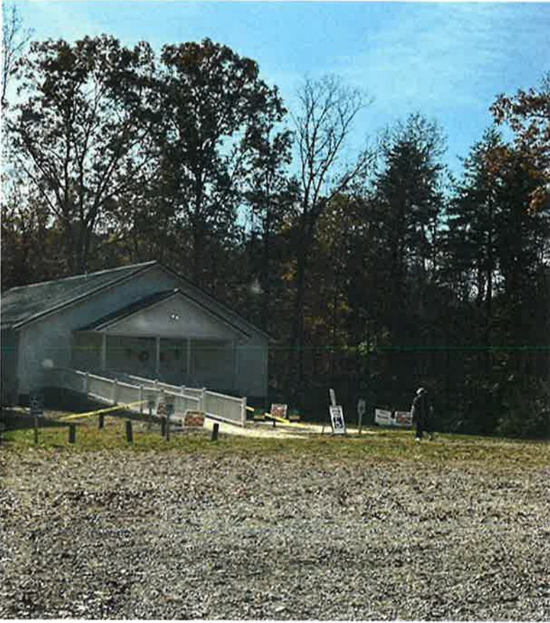
Above: Gravel Lot in Buckingham County. Not clear path of travel to door.
